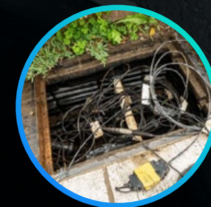
Utility / Service Manholes
